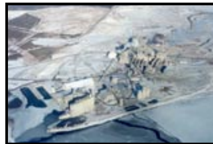
LaFarge Cement Plant Photo credit: Mark Hunter
